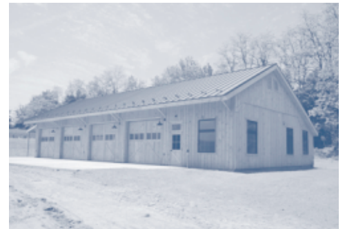
New Equipment Building will house tractors, mowers, and other maintenance equipment
