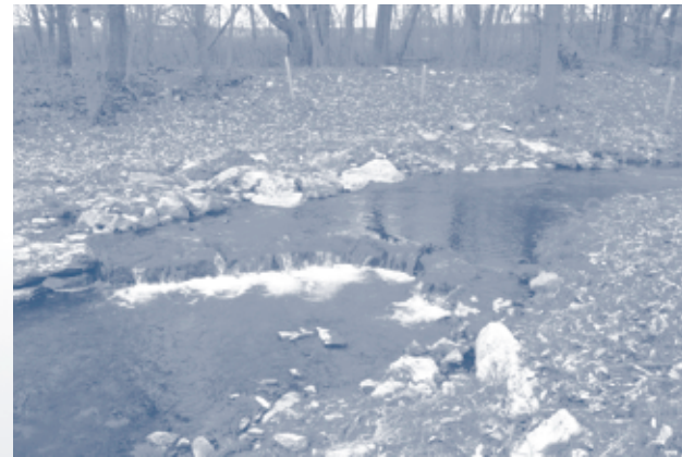
Cross vanes will be one technique used to restore impaired streams
